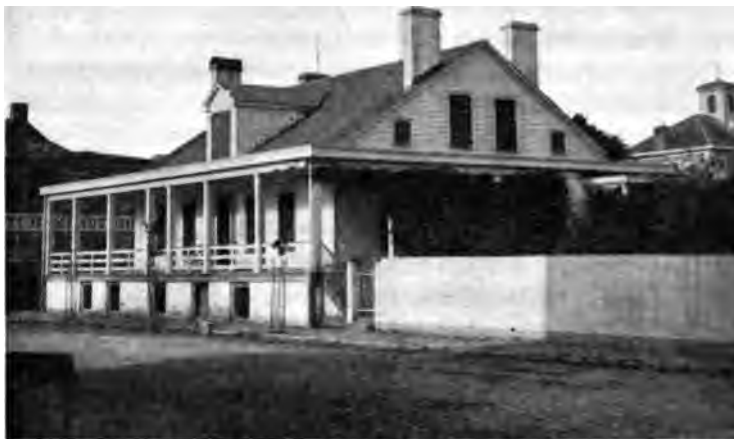
ORIGINAL VALLÉ HOUSE BUILT 1782 -- MODERNIZED
